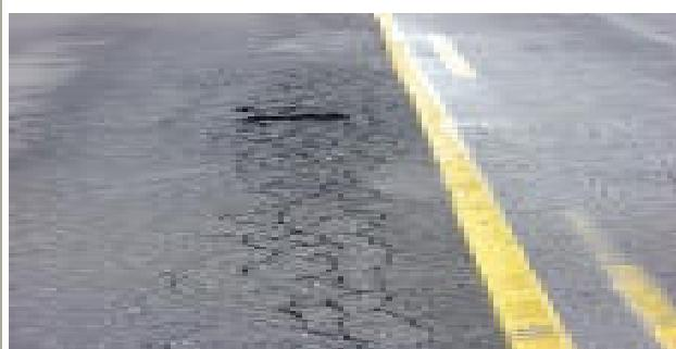
Is there anyone who doesn't know what a pothole is? They can be caused by a number of factors, but usually form when water gets into cracks and destroys the underlying structure. They most often appear when the pavement is most subjected to moisture -- in the early spring.
