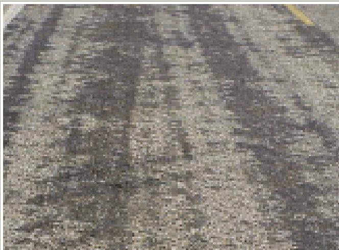
Loose materials (usually aggregate) that "ravel" from the surface or edges of the pavement, resulting in depressions which may fill with moisture and loose aggregate which may pose problems.
