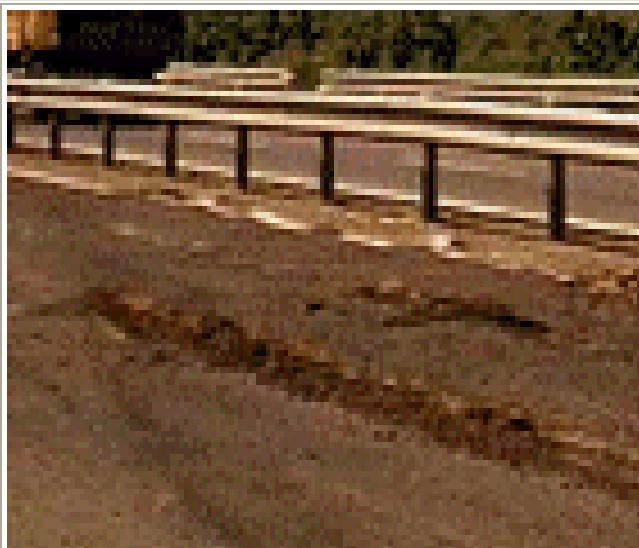
Loose materials (usually aggregate) that "ravel" from the surface or edges of the pavement, resulting in depressions which may fill with moisture and lose aggregate which may
