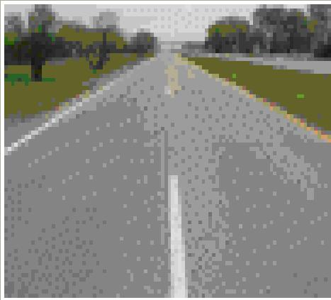
The pavement surface may be a little "dry", is in generally good condition, and is several years old. The underlying structure is also in good condition, showing only minimal visual signs of distress, but it has been subjected to wear and tear.
