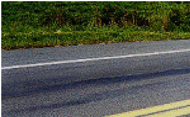
A shiny, black surface caused by liquid asphalt migrating to the pavement surface. The result can mean a loss of surface texture on the pavement.
