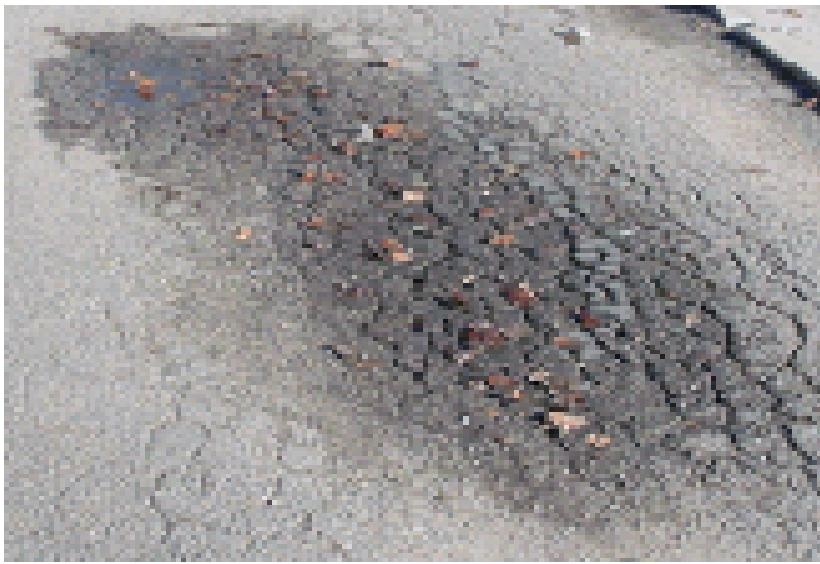
the liquid asphalt binder holds the pavement together and waterproofs the pavement. When moisture gets to the surface of the aggregate it can break the asphalt - aggregate bond, causing the pavement to disintegrate
