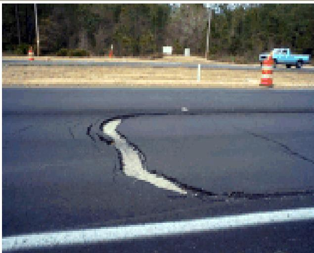
Pushing and Shoving: deformations of the pavement surface, most common in intersections, where there is braking and stopping traffic. It is easiest to detect at intersections where transverse striping becomes "wavy".
